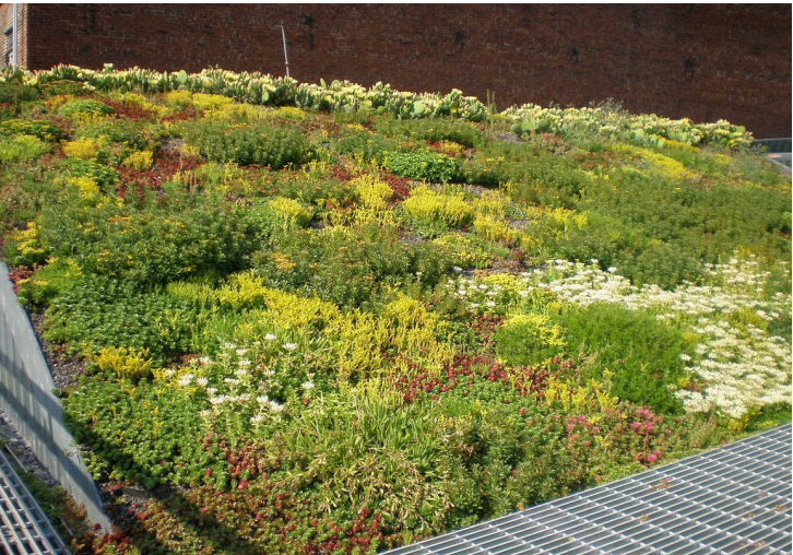
SuDS example – green roof
